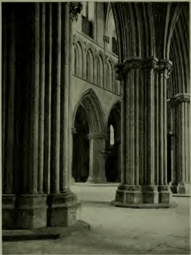
THE NAVE OF WELLS CATHEDRAL FROM THE SOUTH AISLE The Early English clustered columns have capitals enriched with exquisite leaf forms.
